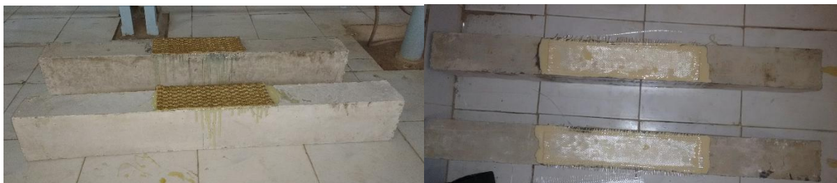
Fig. 4 Beams Retrofitted Using Sisal and Glass Fiber Sheets with Epoxy Binder
